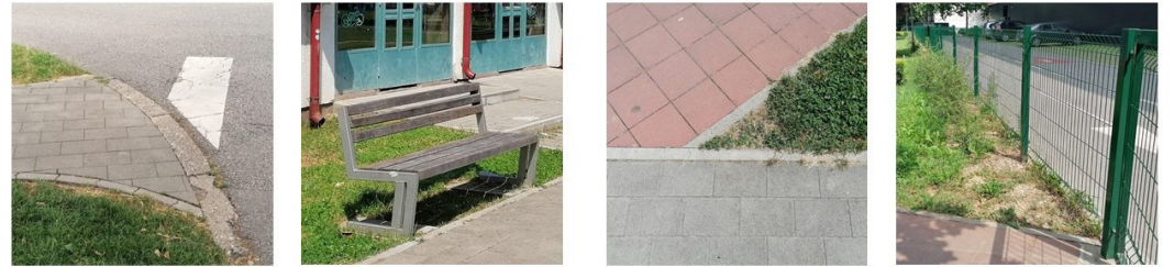
Figure 1: Inclusive design elements. From right to left: gentle slope transition and a marked crossing roads, the legible and familiar design of the bench, alternating tiles to mark different usage zones, a see-through fence to mark ownership zones.
